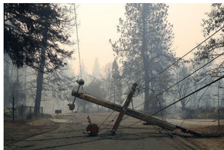
Figure 2 - Overhead telecommunications network destroyed in 2021 in California
